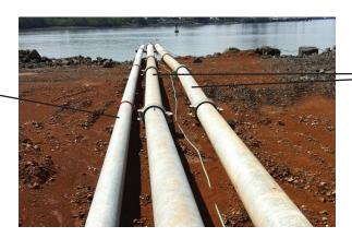
Sphere Lock<sup>™</sup> couplings allow for angled/offset connections.
